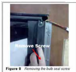
Figure 8 Removing the bulb seal screw
